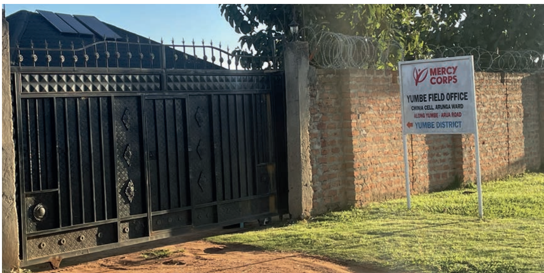
▲ Above: Mercy Corps Yumbe field office
